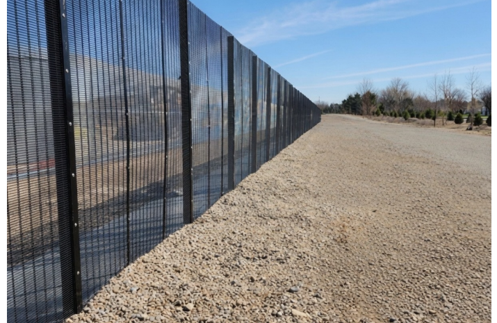
Data-center perimeter — near-transparent mesh for camera and guard observation.
