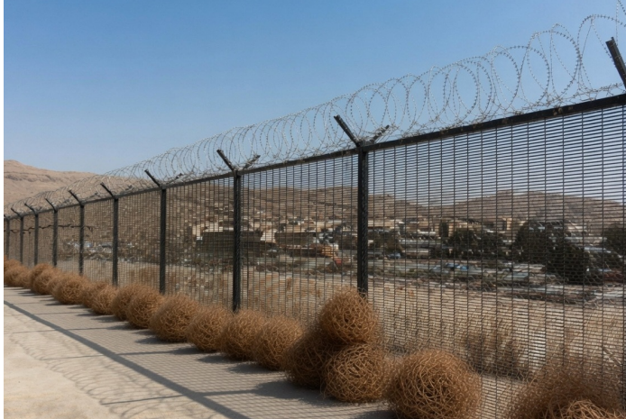
Electric substation perimeter — SecureMesh with danger signage and razor top.
