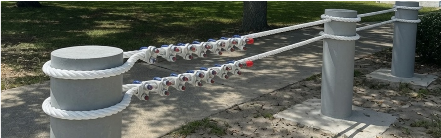
Passive cable line on concrete-filled crash posts at a coastal installation.
