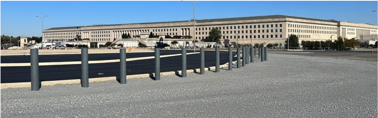
Crash-rated bollard run at a federal facility.
