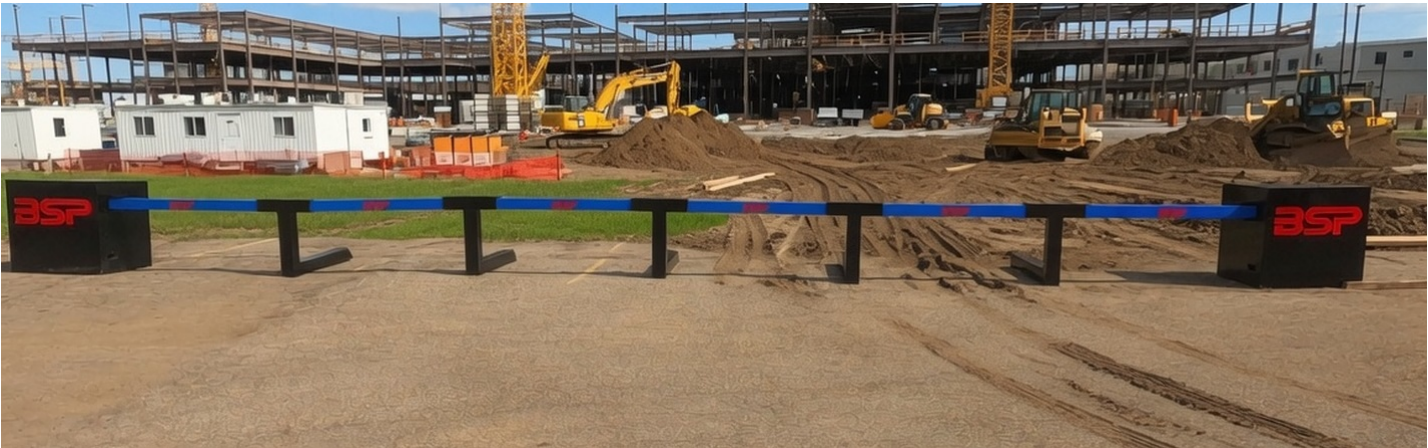
MPPD run securing the perimeter of an active construction site.
