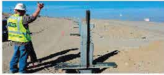
Utah Data Center, Texas
