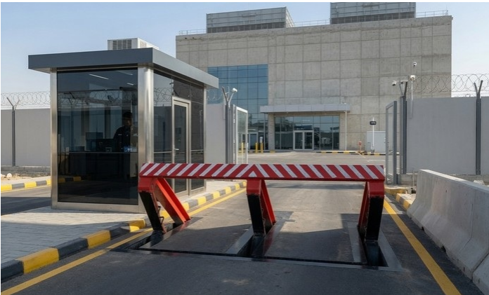
RAL 3020 traffic red with fluorescent striping, deployed at a data-center entry.
