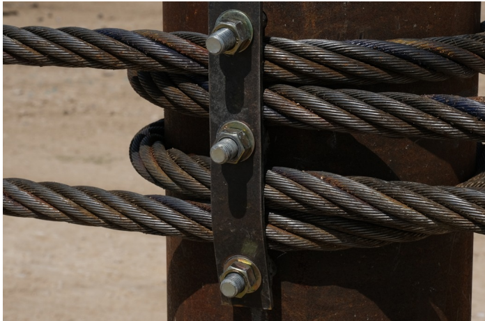
Line crash post after the M50 impact — the cable is wrapped around the post and held by a simple keeper strap.
