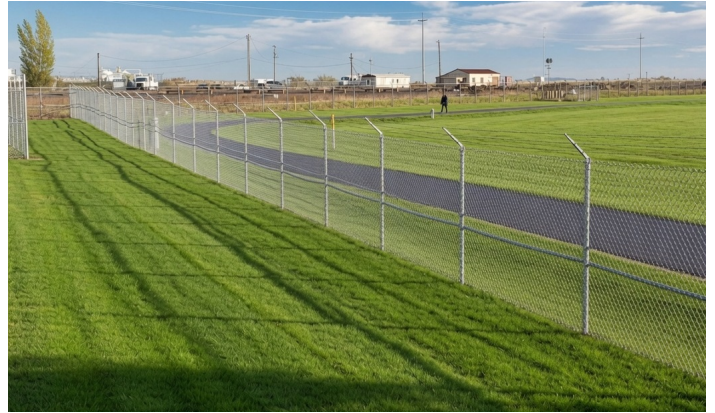
Chain link — Fairchild Air Force Base. Existing fence retained, crash rating added behind it.
