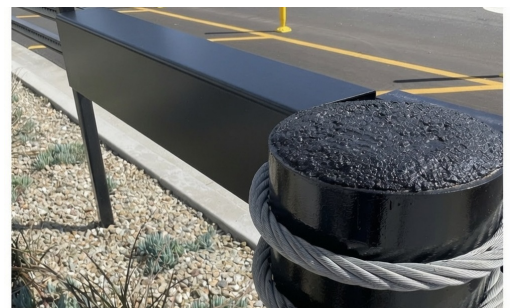
C-channel rail installed over the cable line — the wrapped post carries the rating.
