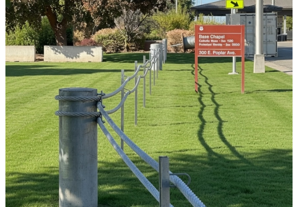
M50 passive cable barrier on a federal campus approach — full crash rating, below sightline.
