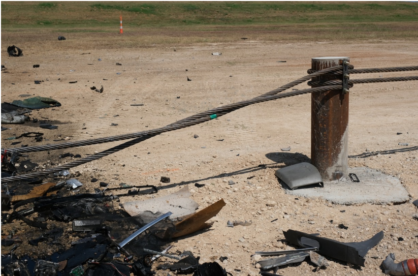
After the M50 test: the crash post is standing, both cables are still anchored, and the truck is the debris field around it.
