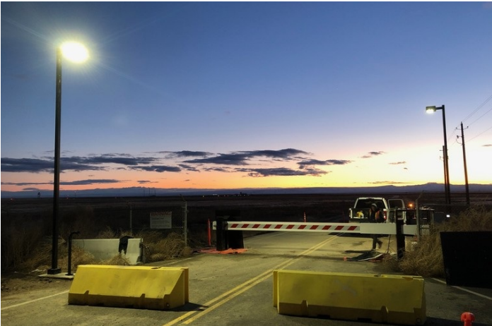
Installation at an entry control point — posts set, beam hung, lane reopened.
