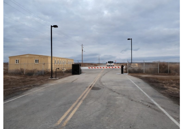
Installed at a controlled entry — both posts on the shoulders, the lane untouched.
