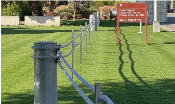
The boundary — BSP Passive Cable Barrier, AVBD 100 Series. M30 and M50, P1 and P2, DoD-listed.
