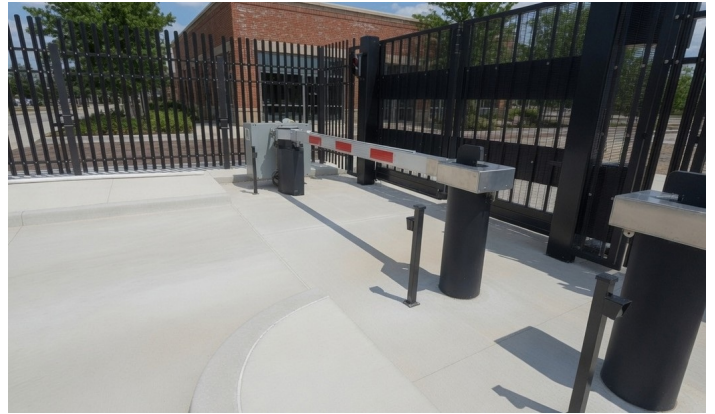
The opening — M30 P1 Drop Arm, AVBD 531. Same Ø36" pier, same auger, same crew.
