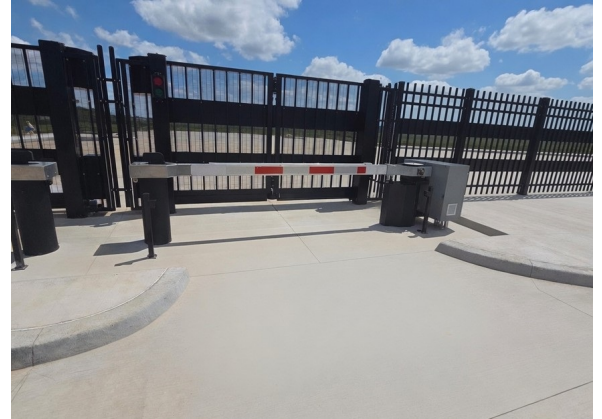
M30 P1 Drop Arm installed at a controlled entry point, shown with the arm lowered.
