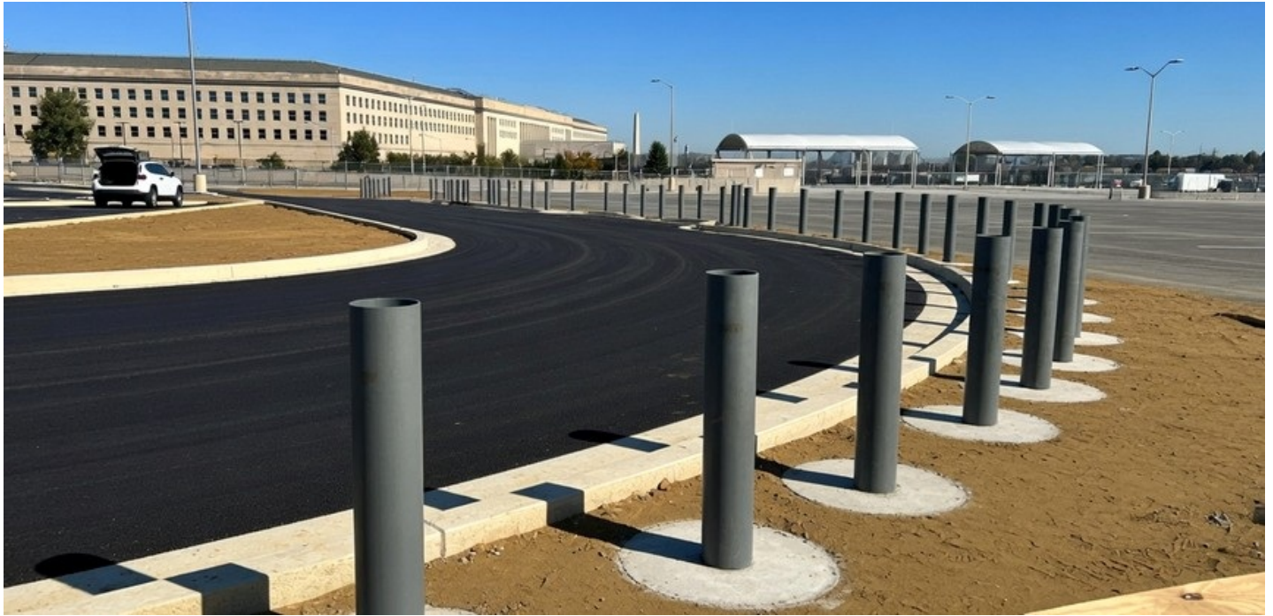
A federal perimeter run mid-installation — pipes standing in finished piers, each one a single circular pour flush with grade, before covers and paving.
