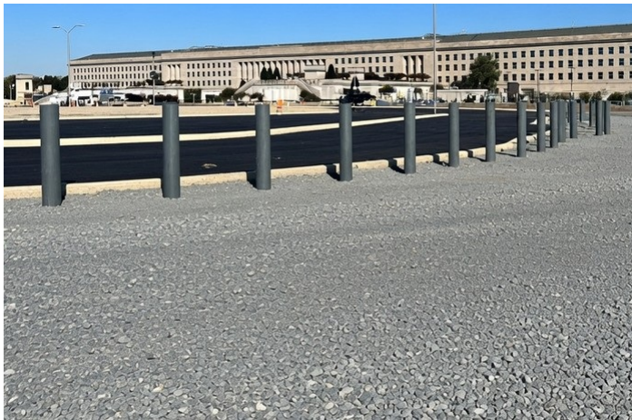
A federal facility perimeter — several hundred feet of rated bollard line along a vehicle approach, in bare primed pipe before covers.
