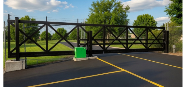
Crash-rated slide gate with chain link infill and a barbed top, on a commercial drive.
